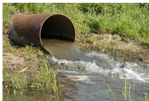
Discharge pipe (source: USAD)
